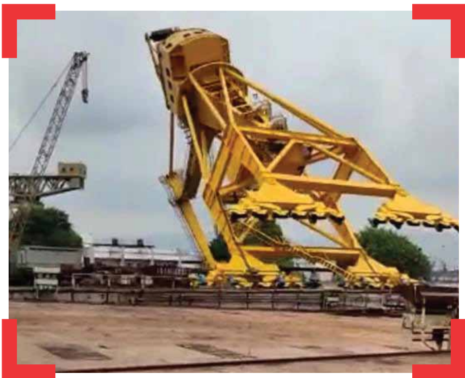
The company did not provide a design manual for the crane, the panel found, and added that four bearings, including central bearings, were damaged, triggering the collapse.
