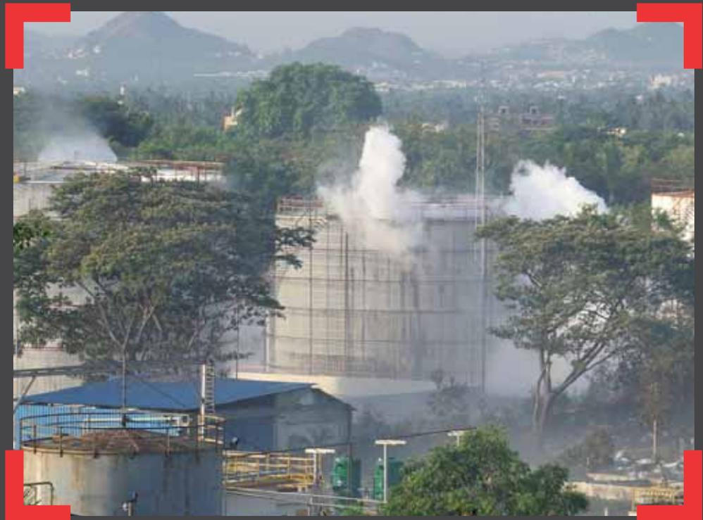
Chiller system was switched off the previous evening as part of routine maintenance and no temperature or pressure monitoring was done at the middle or top of the tank where space is left for vapourisation, found the committee.
