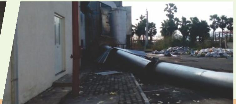
An elastic manufacturing company sustained severe damages to their production facility including their utilities. The collapse of the chimney and related structures affected the production as the utilities supplied steam critical to the manufacturing process. Apart from Material Damage losses, Business Interruption was in excess of 2 months.
