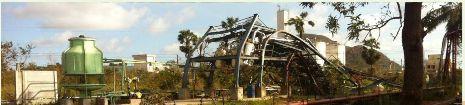
Extensive damages to a Distillation column (Bent/ Twisted/ Damaged) in a chemical factory. The losses were estimated at more than Rs. 7.5 crore, including damages to buildings and other equipments.
